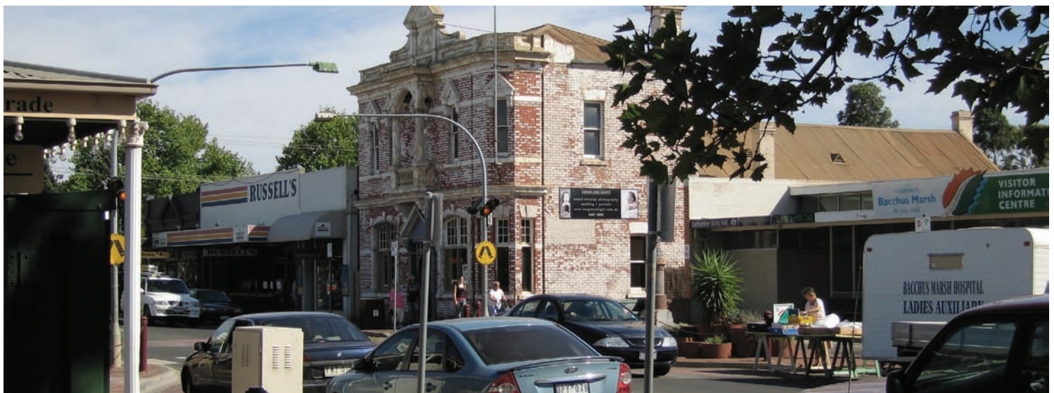
Bacchus Marsh main street. Strategy prepared by THA Landscape Architects for Moorabool Shire Council
