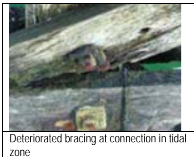
Photograph 3: Condition of bracing
