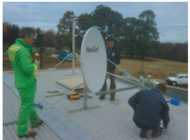
James Milner of SII (left) helps set up the GPSnet base station on the roof of the Kinglake recovery centre
